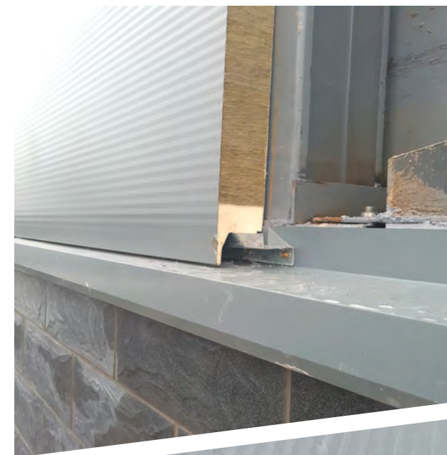
Joint with gap for horizontal application
