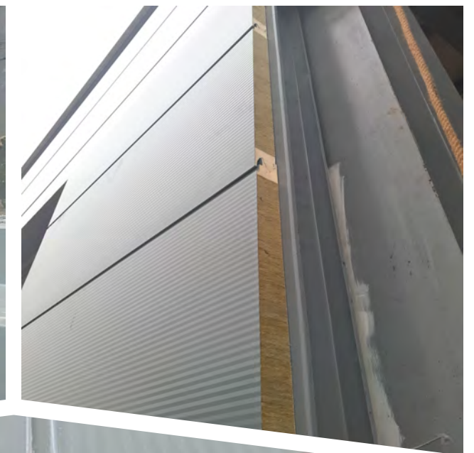
Joint without gap for horizontal application
